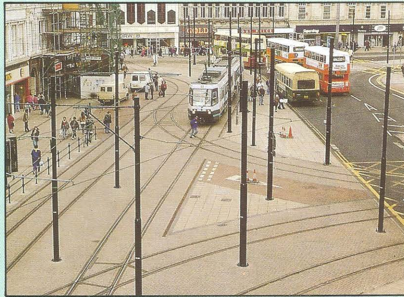
The "delta-junction" in Piccadilly is the focal point for Phase 1 of Metrolink and also for the planned extensions.
