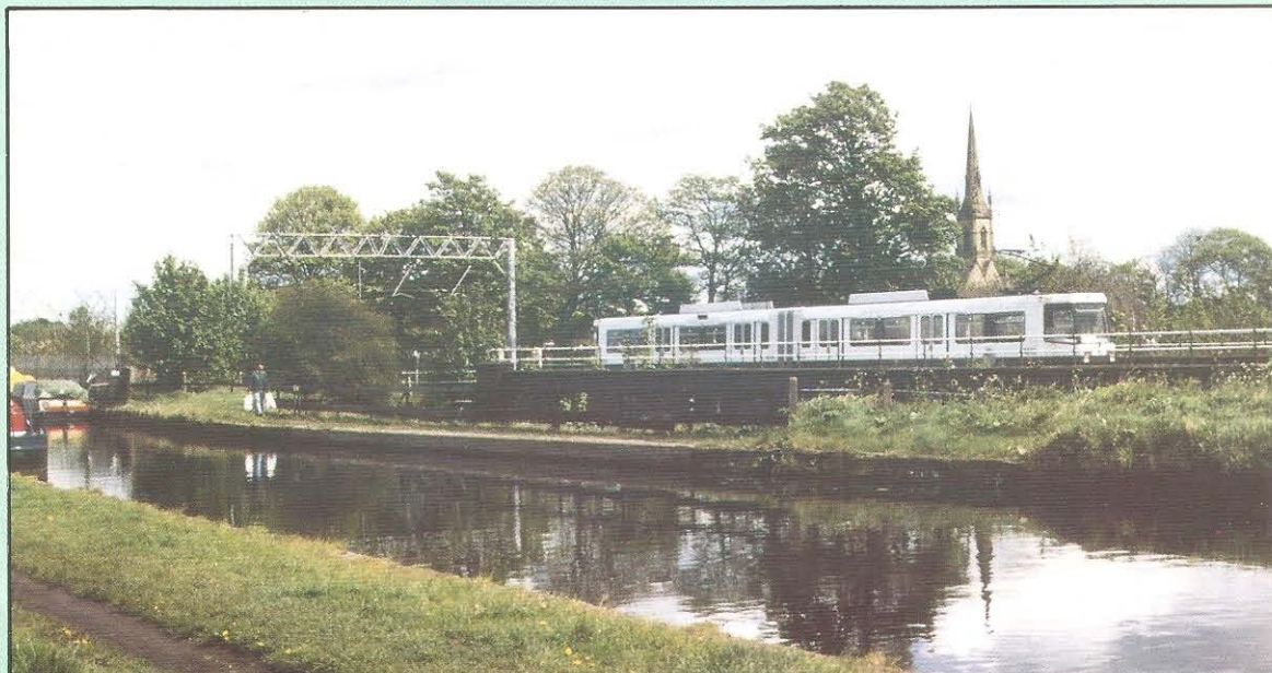
(Above) The Bow-string bridge was designed to complement the style of the nearby G-Mex Centre. The adjoining viaduct is actually of concrete construction but is faced with factory-assembled
